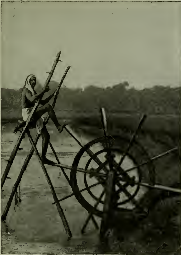
Here is another curious way of raising water by treadmill which is often practiced in India.
